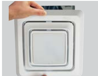
Attach new fan cover
